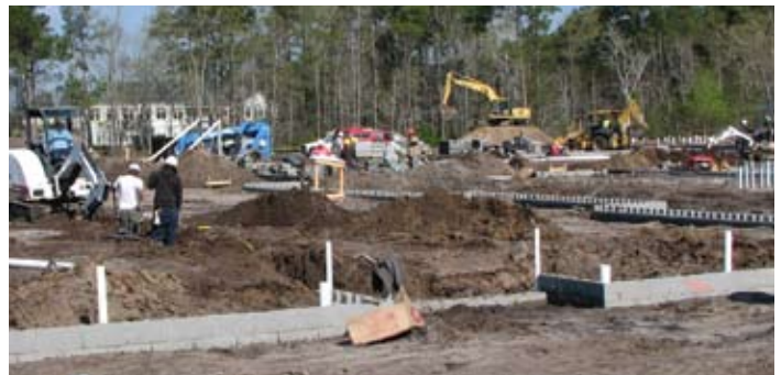
Wilmington construction, March 2010
